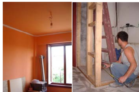
The renovation has started
